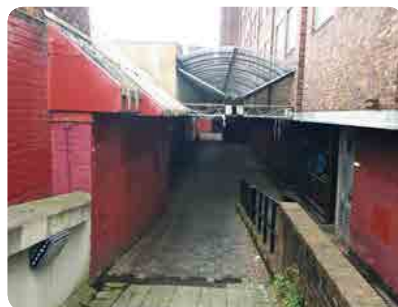
[Premier Inn - poor pedestrian access to bridge link]
