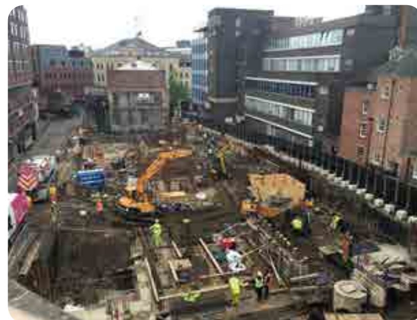
[Student accommodation under construction]
